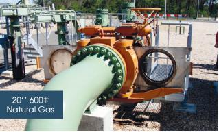
During the commissioning of a sectioning station, a 3 positions slide gate with calibrated orifices is used to ease the flush out of the pipe filled by air.
